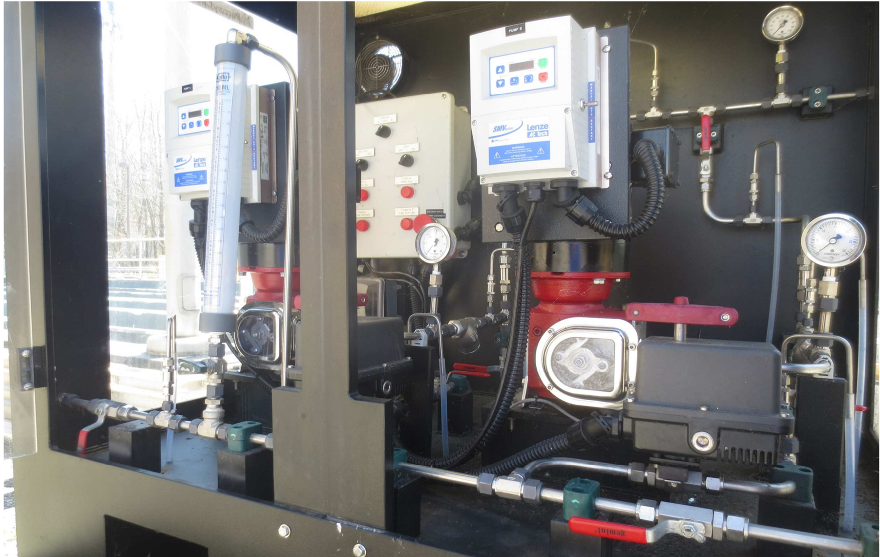
Mt. Holly MUA Peracetic Acid Dosing System (temporary)
