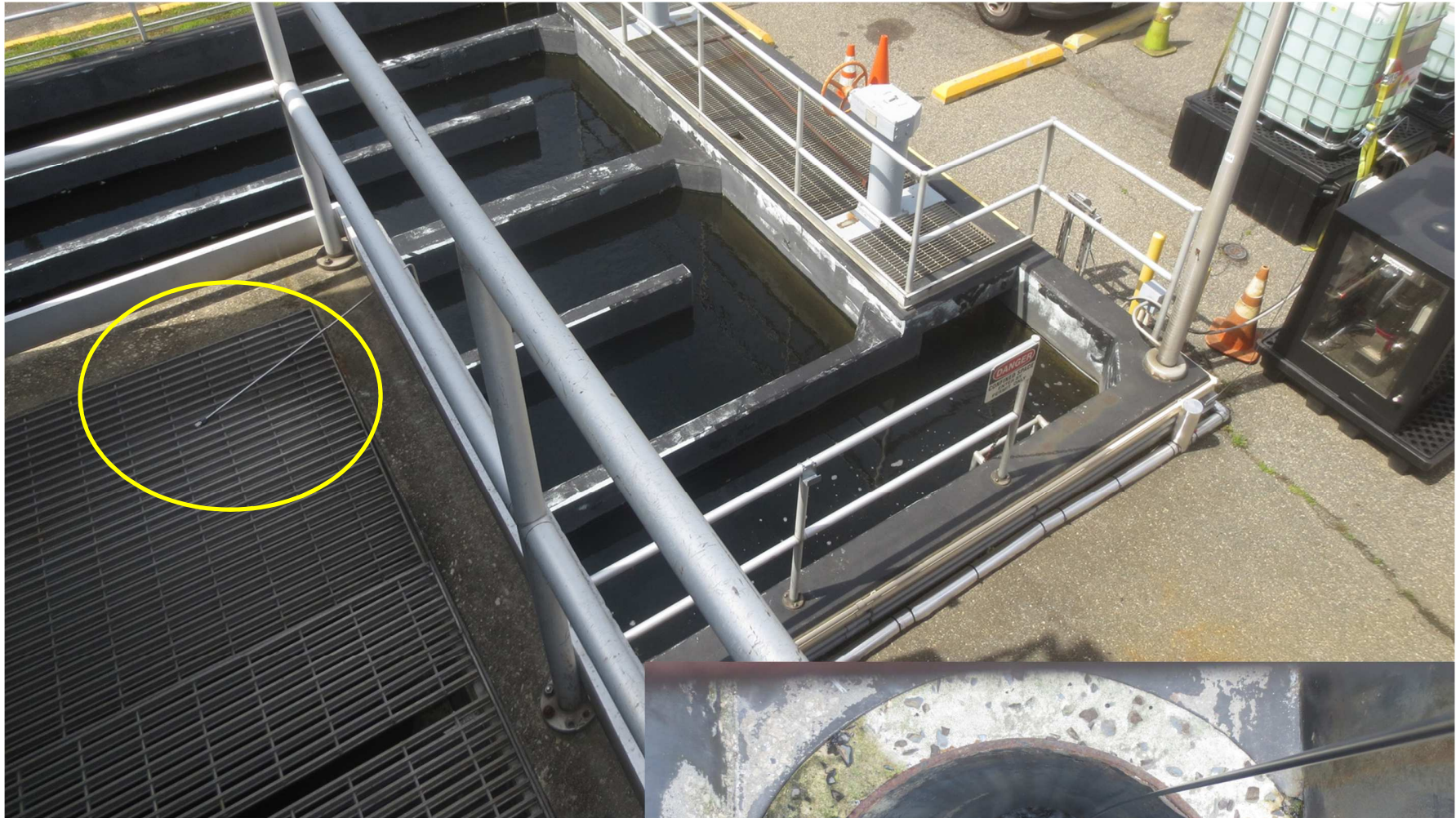
Mt. Holly MUA Peracetic Acid Application Point (temporary) 1/8" 316L SS Tubing
