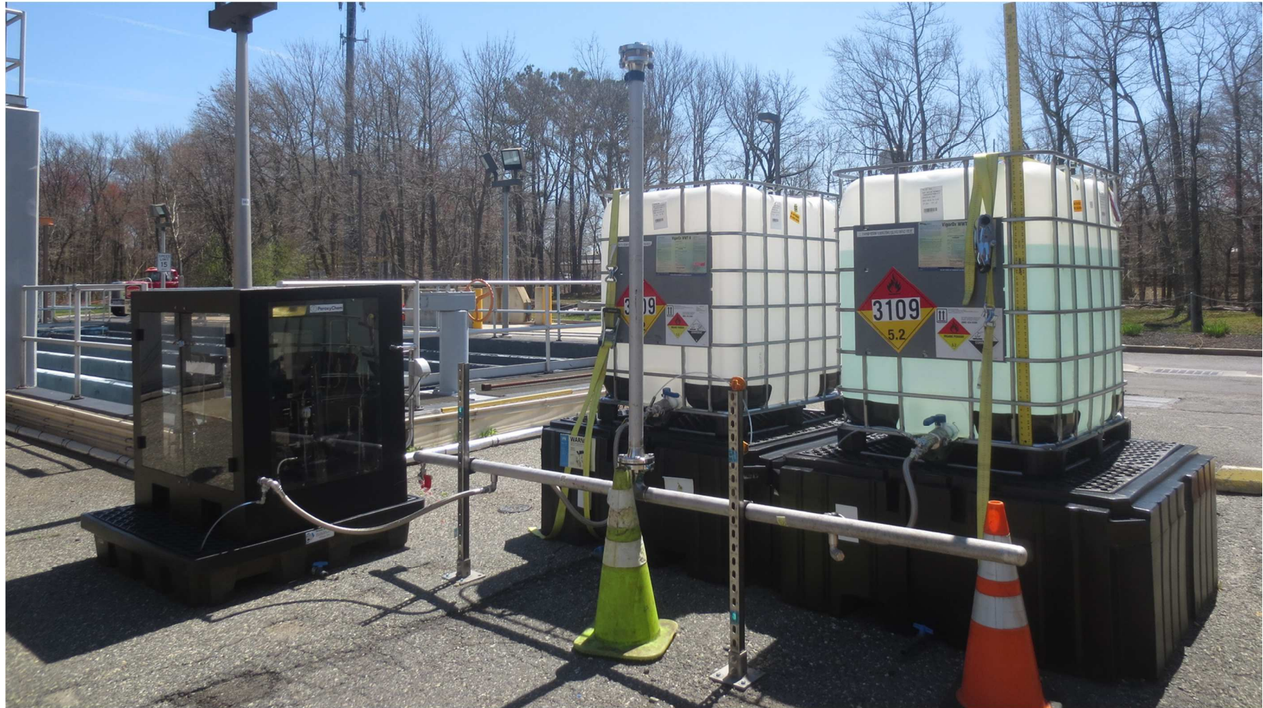
Mt. Holly MUA Peracetic Acid Dosing System (temporary)
